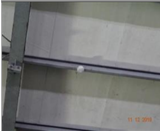
External photo(s) of the production unit(s) Smoke detector had been equipped.JPG
